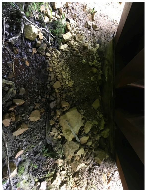
Left Bank Abutment when facing downstream
