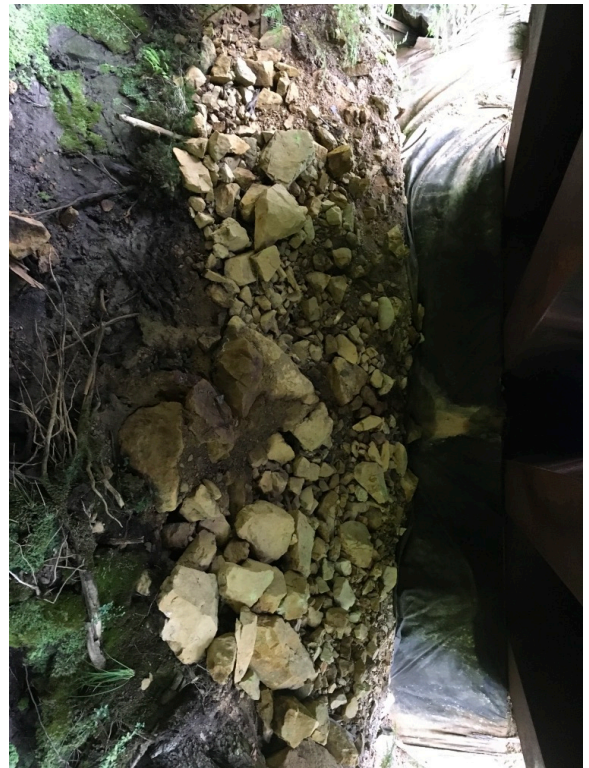
Right Bank Abutment when facing downstream
